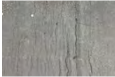
Asphalt Cracks
